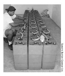
Fig. 7.2: Deep-Cycle Lead-Acid Batteries. These batteries contain thick lead plates and are used in many batterybased renewable energy systems. The thick plates permit deep cycling so long as the batteries are recharged soon after each deep discharge.
