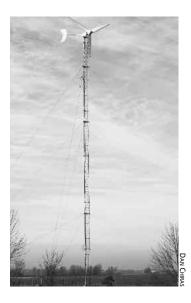
Fig. 1.3: Small Wind Turbine on Tower. This ARE442 wind turbine installed at Mick's house is mounted on a guyed lattice tower. Maintenance is performed by climbing the tower.
