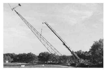
Fig. 6.5: Crane Lifting Tower and Turbine. This 80-ton crane lifts a massive turbine and tower into place. The hinges at the base of the tower allow the crane to tilt the tower into position.
